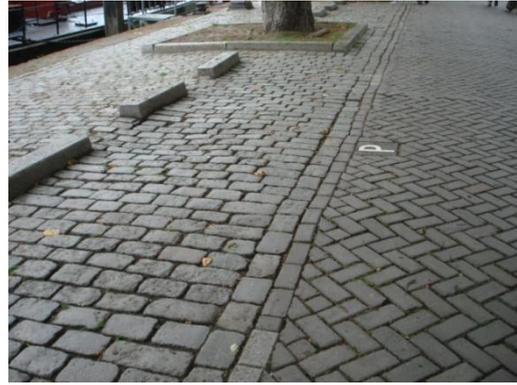
Figure 7 A short kerb can be less intrusive than a bollard - as here in the Netherlands
