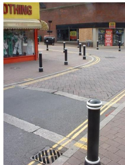
**Figure 3 Bollards used to protect pavements and keep vehicles clear of the footway where there is a low or no kerb**
