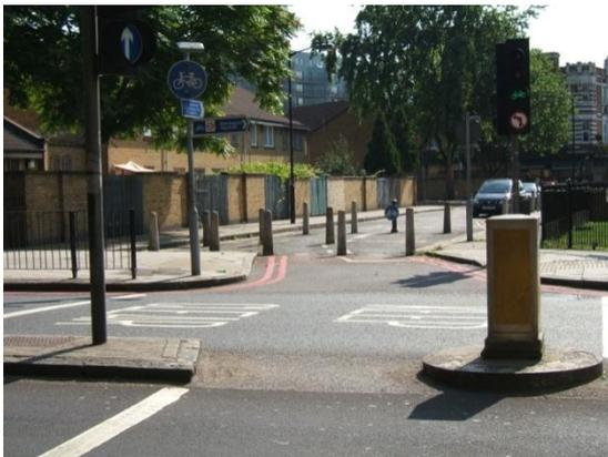
**Figure 1 An incorrect used of multiple bollards - a temporary traffic device that has become permanent**
